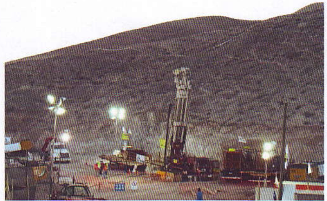
"The Miracle" in action drilling the rescue shaft
